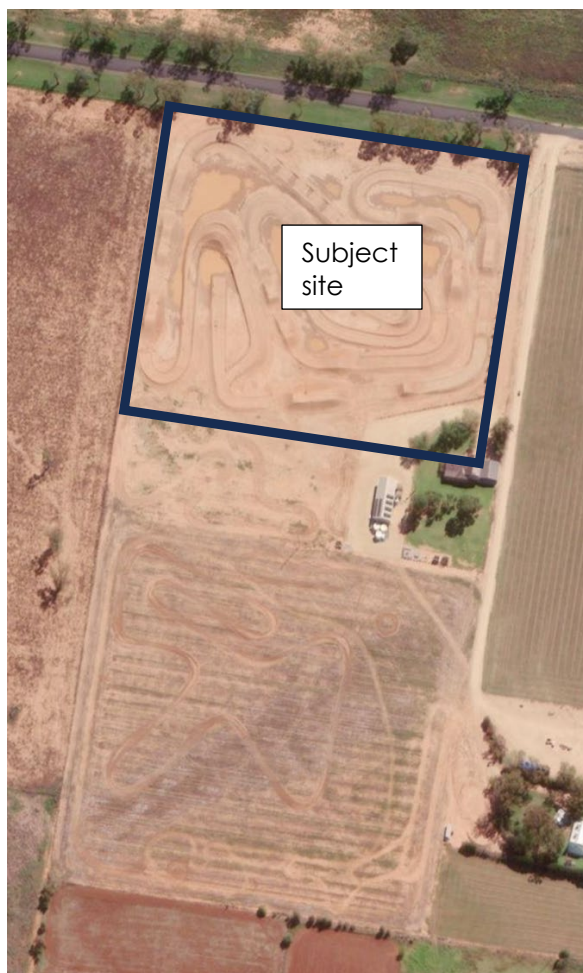
Figure 3: Aerial close view of site showing earthworks
